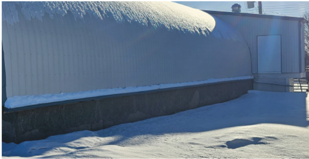
Photo 8. Foundation– West side
