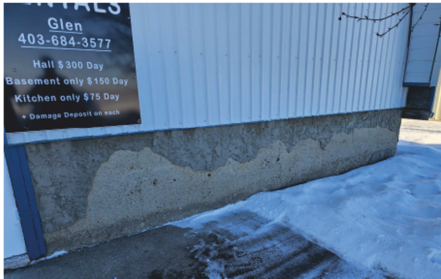
Photo 7. Foundation– North side
