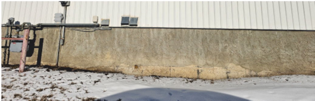
Photo 9. Foundation– South side
