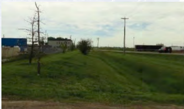
Roadside ditching for stormwater conveyance
