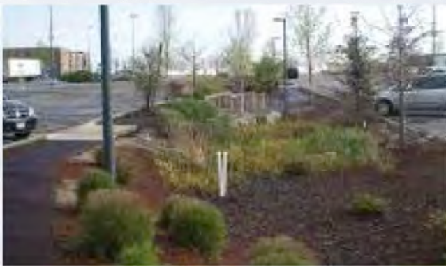
Vegetated drainage swale
