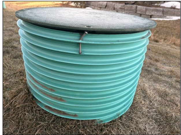
Figure 3.2: Damaged Bolt
